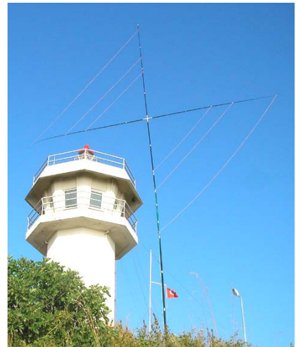
1ele Quad 20/15/10 am 12m Fiberglasmast
